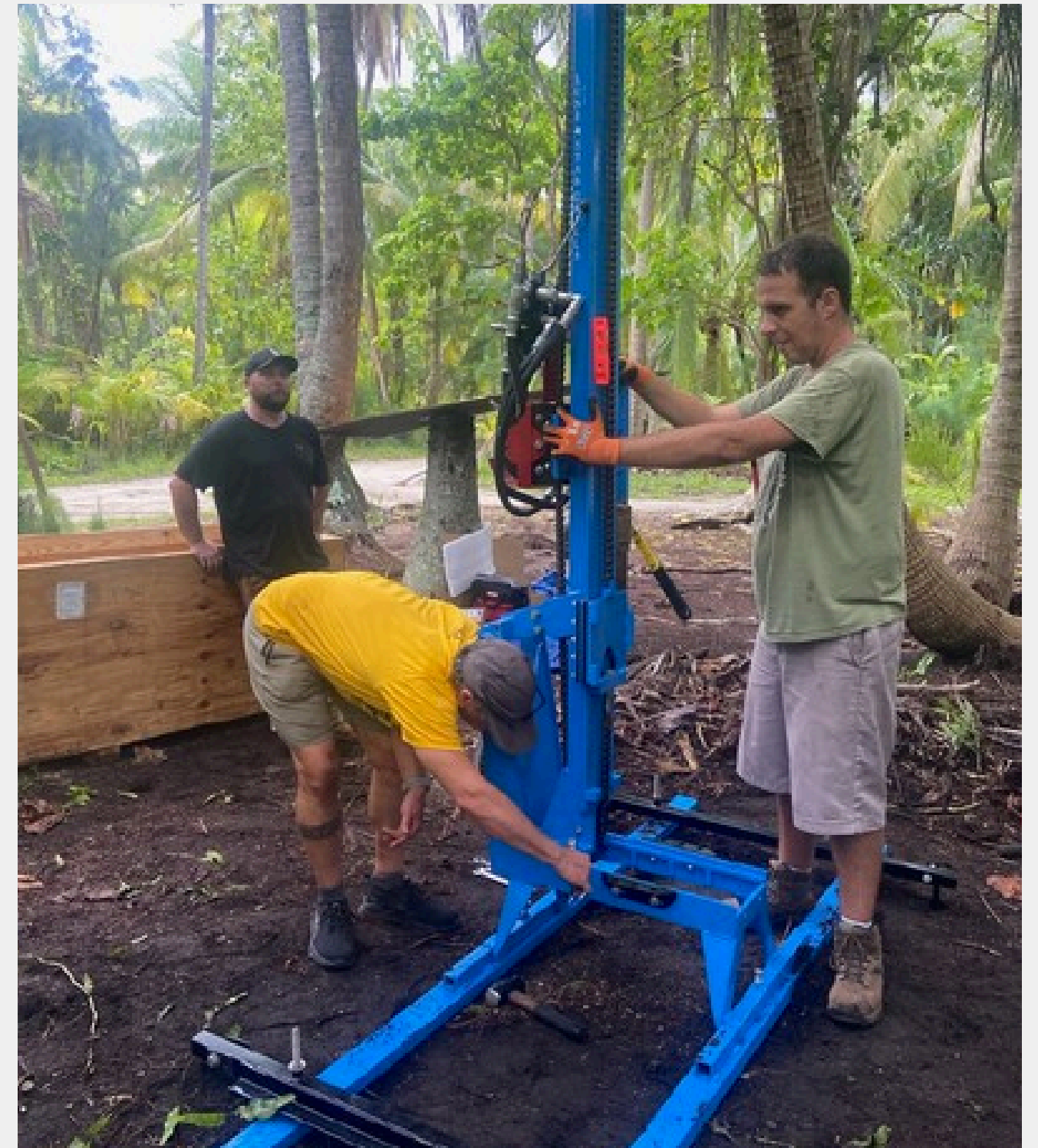
Installation of a piezometer for groundwater studies
